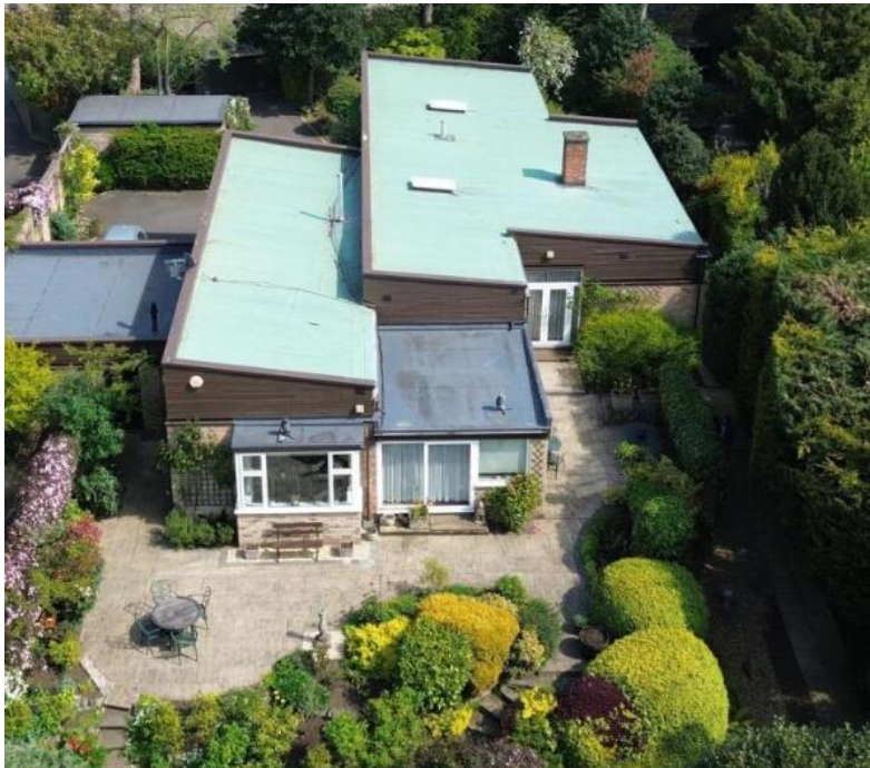
Aerial view from rear
